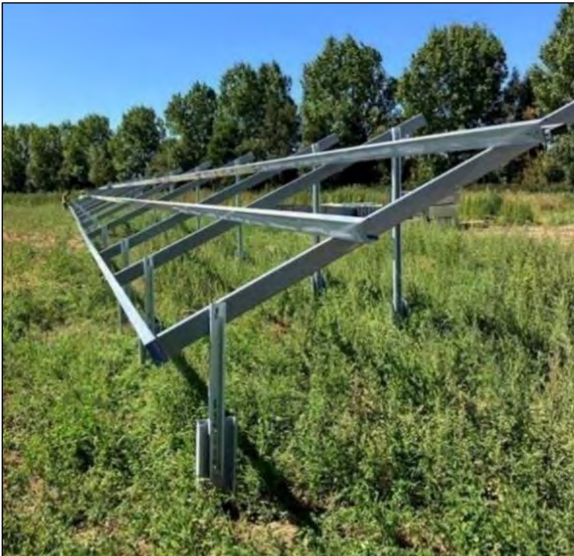
Plate 2.10 Typical Solar PV Module Mounting Structure installation
